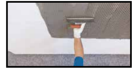
Spread the adhesive using a notched trowel vertically
