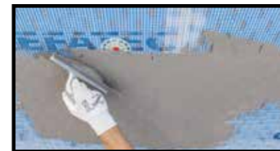
Smooth and fill the mesh with a notched trowel in a vertical direction
