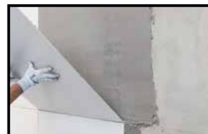
Bonding of ZERO.3
