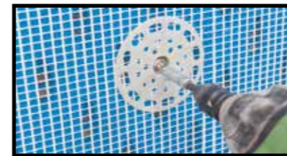
Place anchors: at least 5 per m 2
