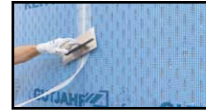
Apply Watec ST - joint netting
