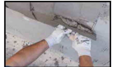
Second layer of PLANITOP HDM MAXI
