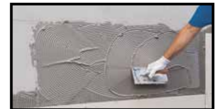
Double buttering (on wall)
