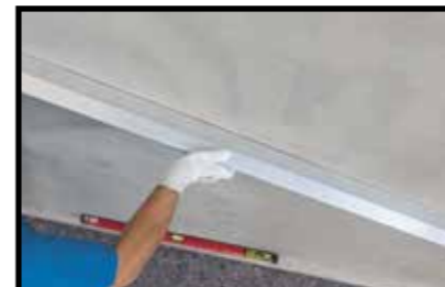
Control the flatness of the structural plaster
