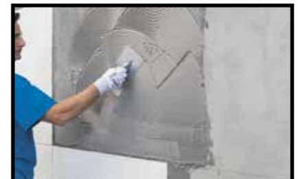
Double buttering (on wall)
