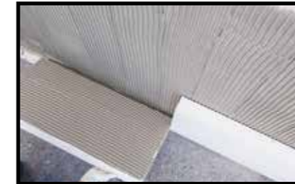
Installation of insulation panels with double buttering
