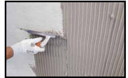
Installation of insulation panels with double buttering (on wall)
