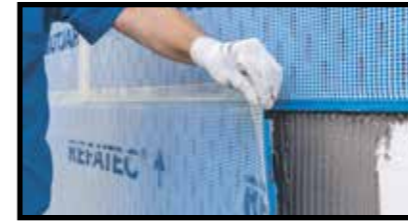
Lay CeraVent matting from top to bottom, alternated
