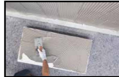
Installation of insulation panels with double buttering (back of tile)
