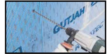
Place anchors: at least 5 per m 2
